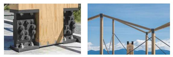
Figure 4. Implementation of the RSFJ technology in the new airport terminal, Nelson, New Zealand
